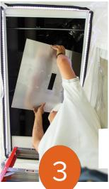
Each CAP model installs easily and lays flat and flush with ceiling grid with the protected opening facing down toward the floor and rollers facing the ceiling.
