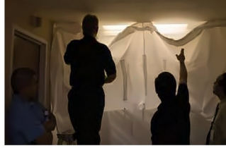
Corridor flange deployed in place
