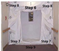
Install order: ceiling (6), walls (7-8), floor (9)
