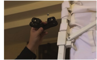
Install a structure support on the frame
