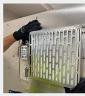
Embedded, adjustable speed negative air machine with prefilter and HEPA Filter.
